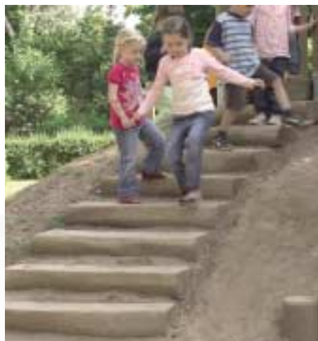
Steps without retaining stakes
