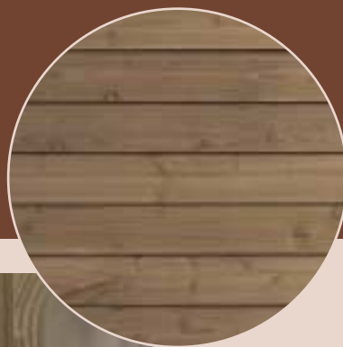
Mitered lapped planking, horizontal
