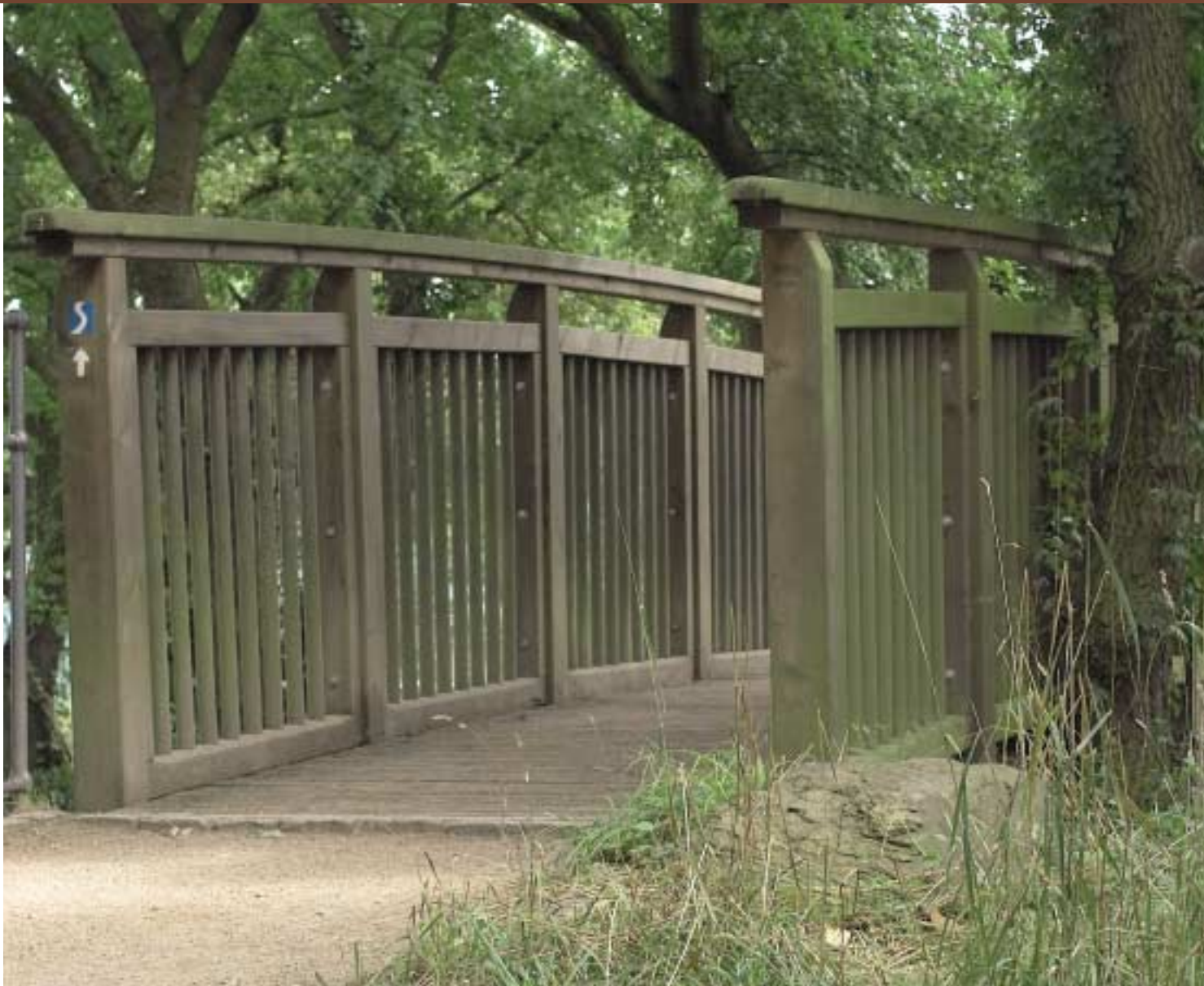
Smart construction and design suited to the landscape -- "Made by HOMBACH". Our company manufactured and built this special wooden bridge, which was installed on the plateau of the Loreley crag It bridges a ravine on the storied cliff and gives visitors a view of the breathtaking Rhein panorama.
